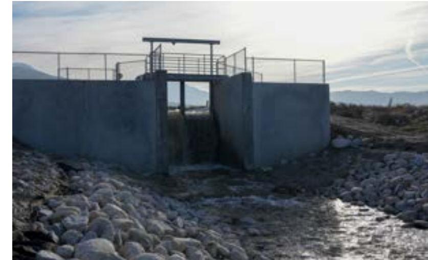
Drop structure at the Enhanced Recharge Project slows water flow to reduce energy and minimize channel erosion.
