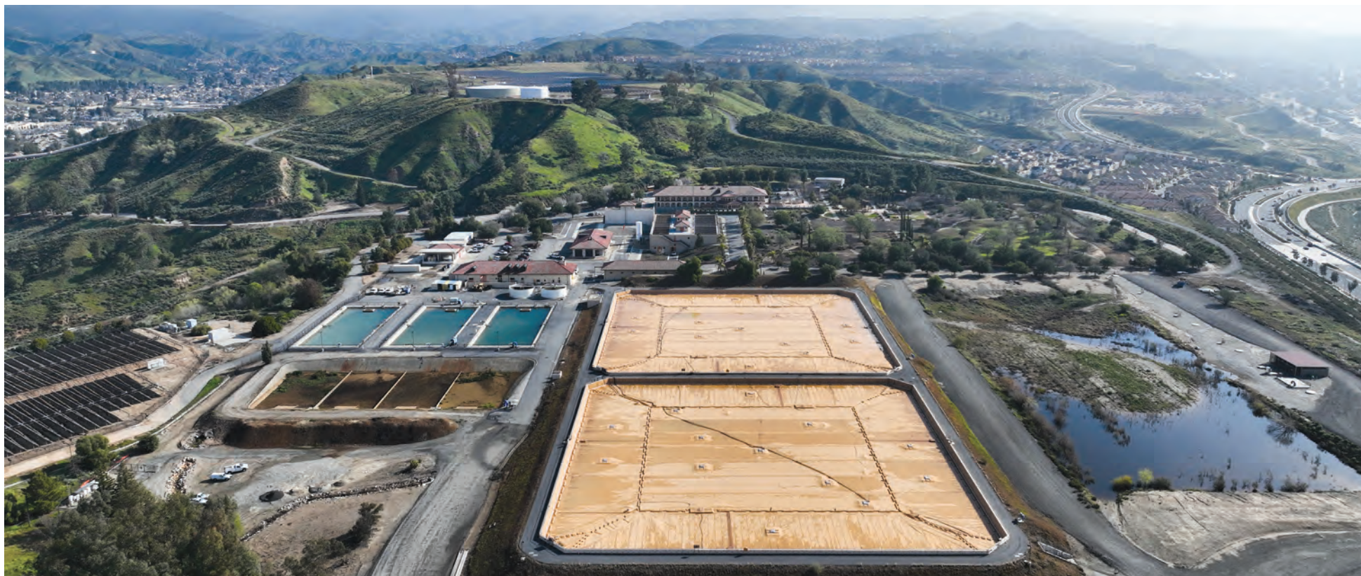
A drone image of SCV Water's Rio Vista Water Treatment Plant with a view of the Santa Clarita Valley.
