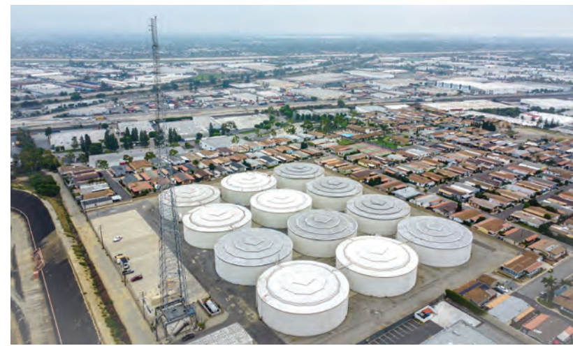
These potable water tanks at J. Will Johnson Reservoir provide imported Metropolitan water to approximately 25% of the city. Long Beach's two drinking water reservoirs, J. Will Johnson Reservoir and Alamitos Reservoir, sit at the same elevation, working in tandem to optimize water quality management and maximize energy efficiency – using gravity to distribute water to the entire City of Long Beach.
