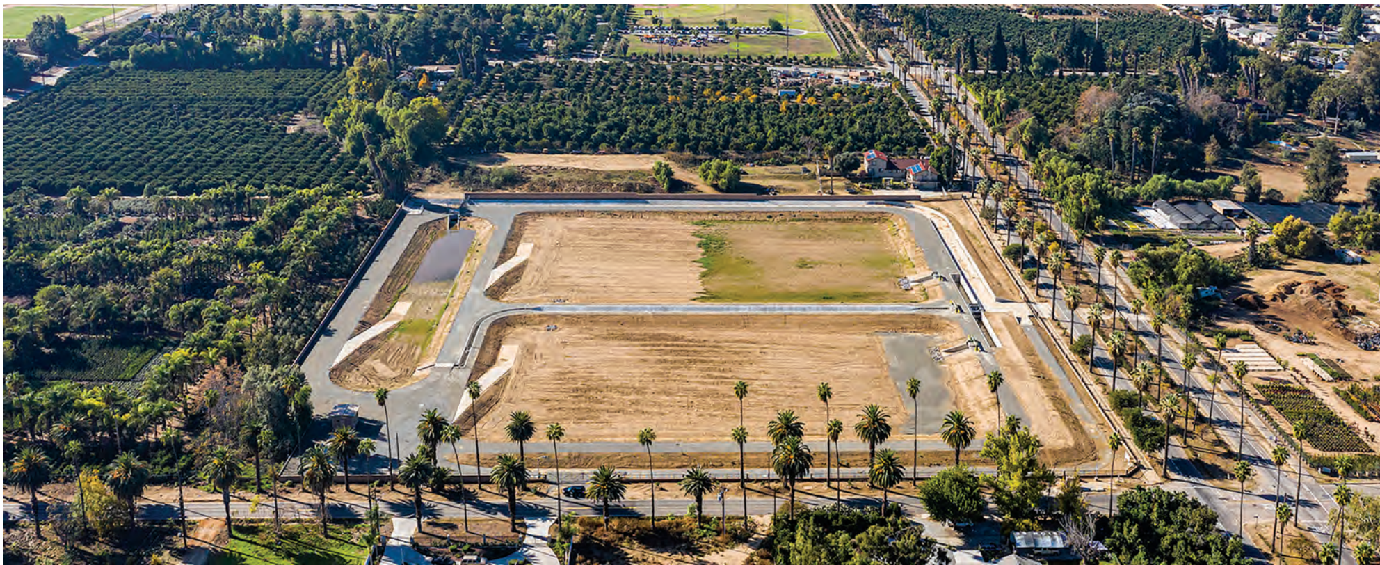
Completed in early 2021, the Victoria Recharge Basin is a strategic part of Western's plan to develop local, reliable water supplied for the region and is designed to capture stormwater runoff to allow it to seep into the groundwater aquifer below.
