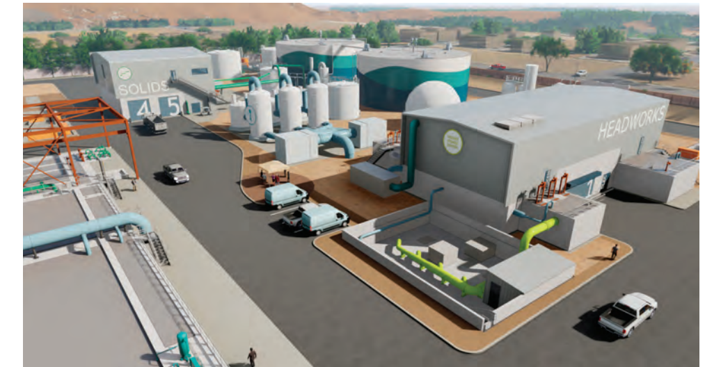
Top, EVWD General Manager/CEO John Mura looks over construction of the Sterling Natural Resource Center in Highland, which will open in 2022. The SNRC, as shown in the rendering above, will include a wastewater recycling facility as well as co-digesters that will convert organic waste into electricity.
