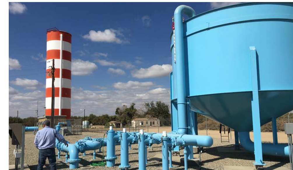
Semitropic Water Storage District facilities in Wasco, in Kern County.
