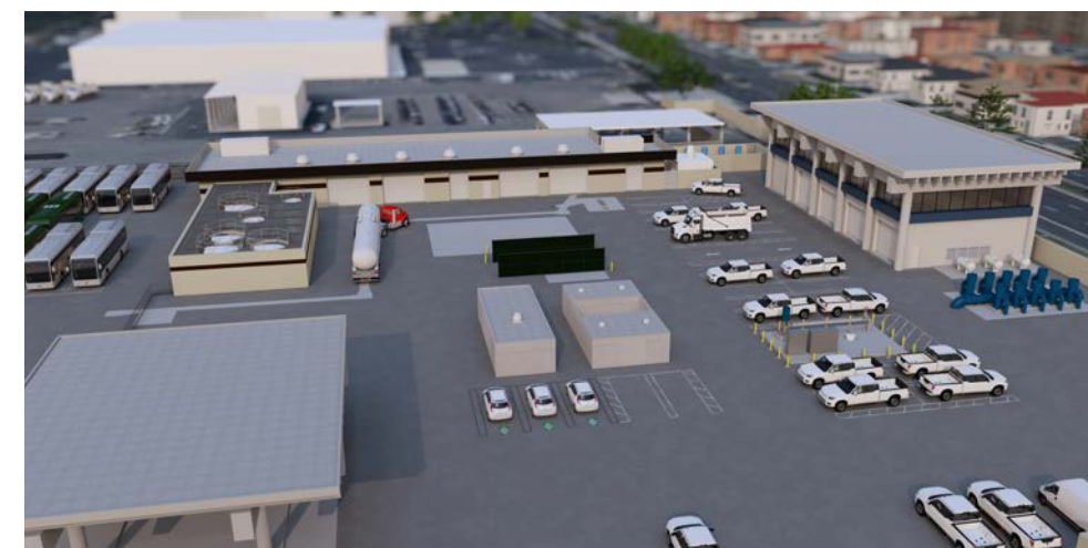
An early rendering of what the expanded Torrance Groundwater Desalter may look like. The expanded facility will include additional pretreatment and reverse osmosis as well as automated strainers to protect the reverse osmosis systems.
