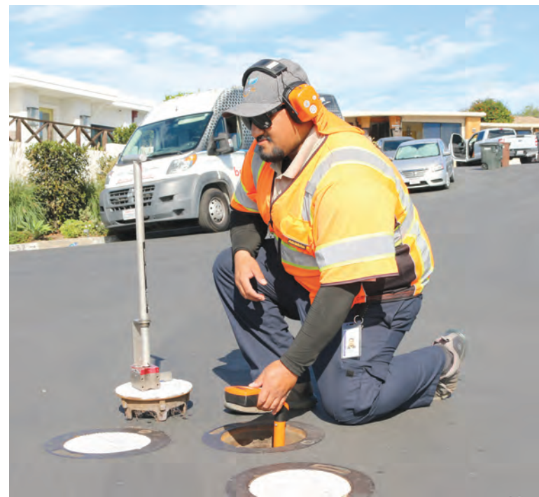
MWDOC leak detection technicians use listening equipment to find hidden leaks.
