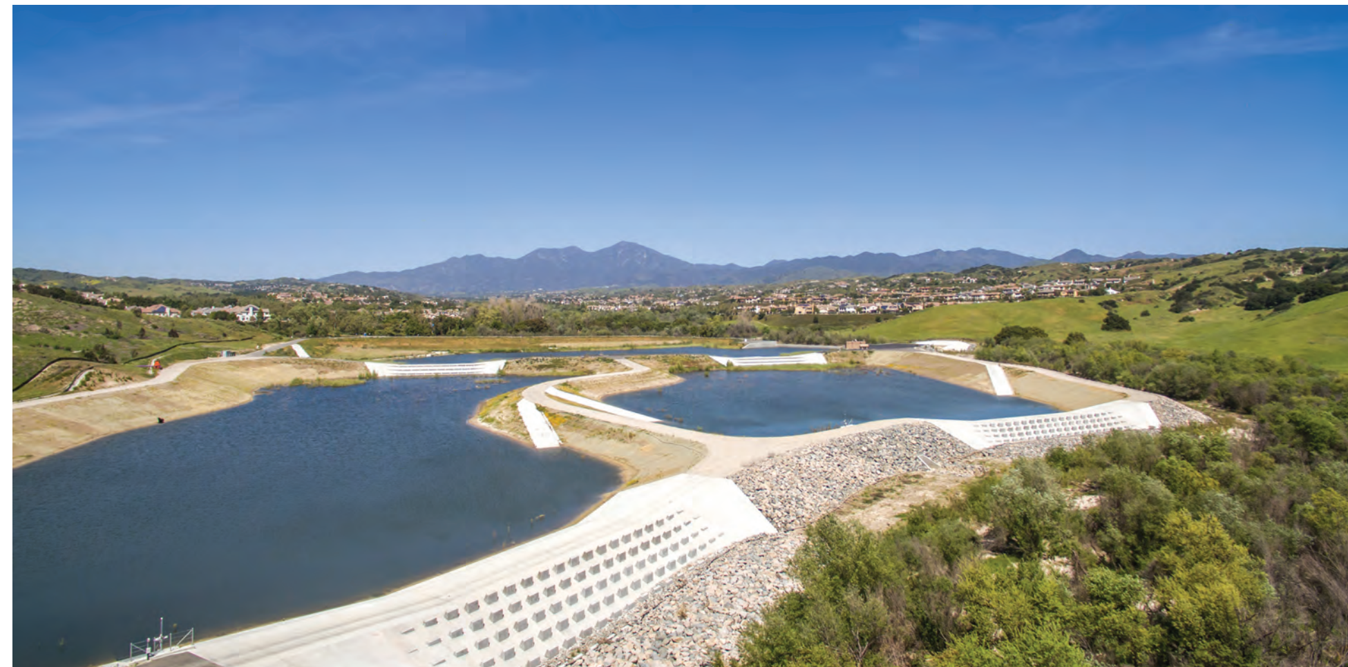
Santa Margarita Water District’s Gobernadora Multipurpose Basin south of Cota de Caza, shown above and at left, captures and naturally treats urban runoff and storm flows, and uses the urban return flows to help meet irrigation demands in the nearby community. At right, Upper Oso Reservoir stores recycled water for use during hot, dry months.
