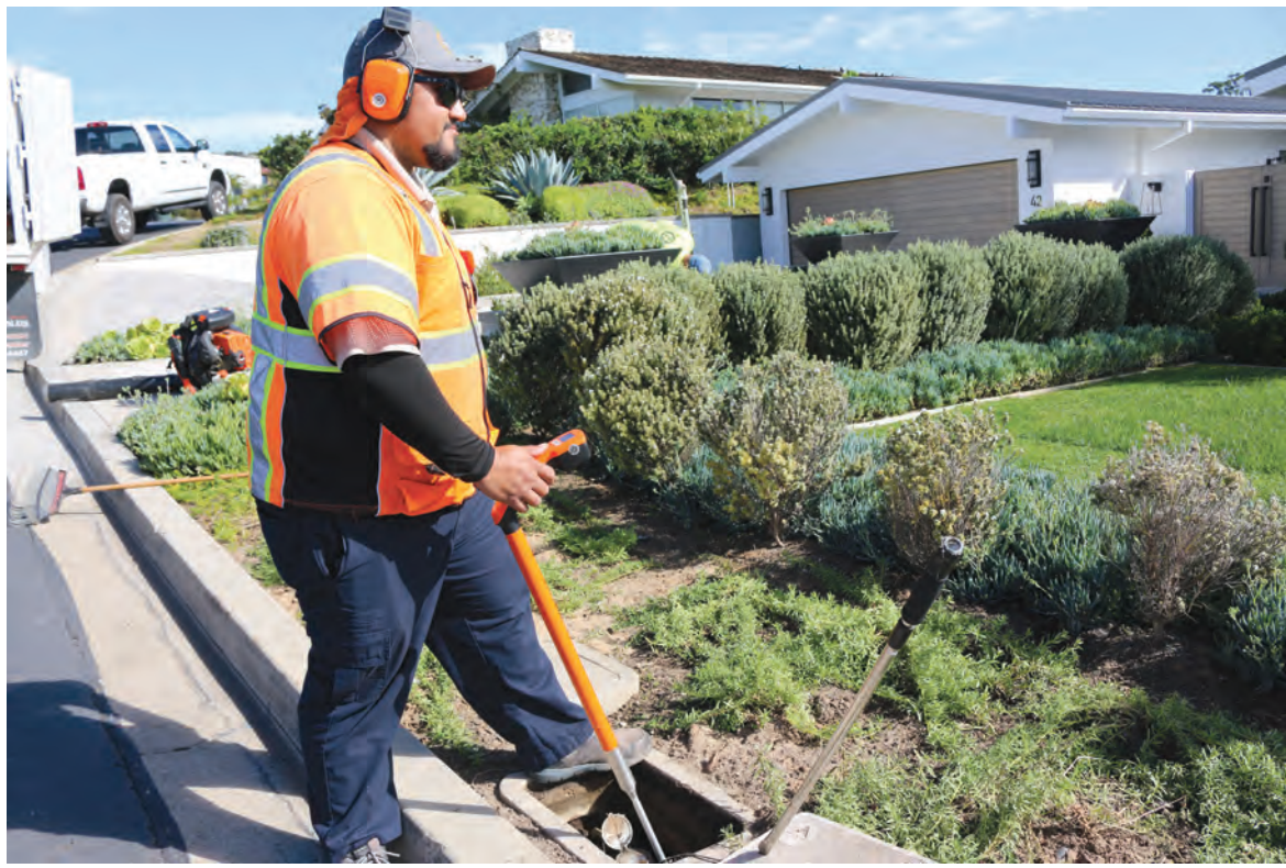
MWDOC leak detection technicians use listening equipment to find hidden leaks.
