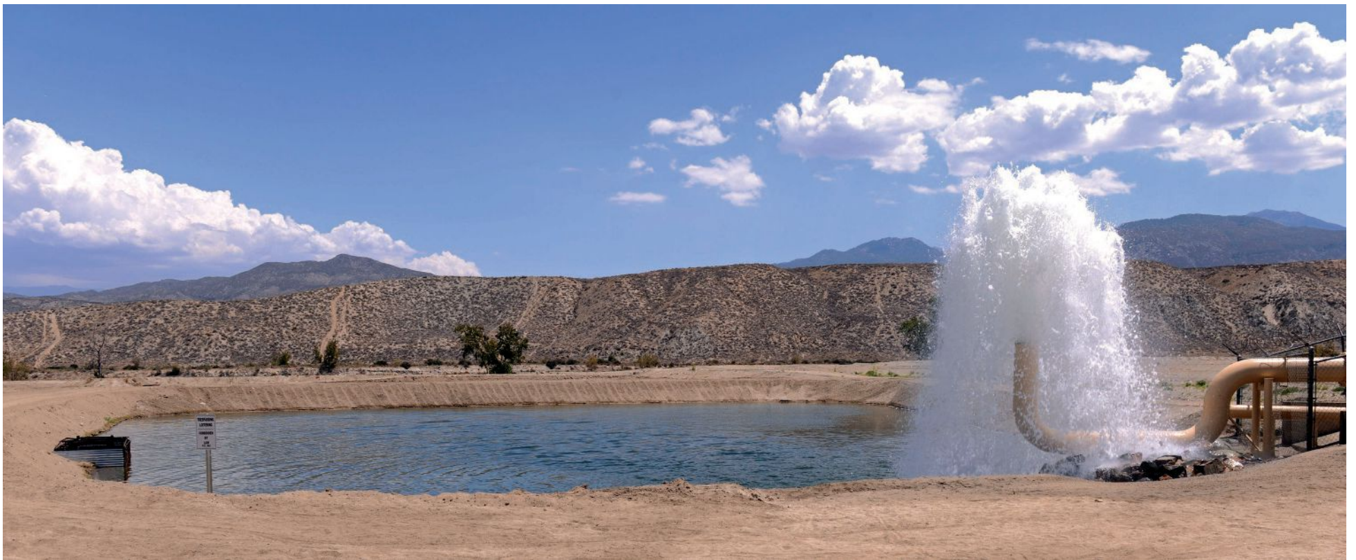
EMWD replenishes groundwater in the San Jacinto Valley during wet and normal years so that it has an increased supply of local groundwater supplies available during cyclical dry conditions. Below, EMWD uses recycled water for public landscaping, including at golf courses and in common areas of homeowners associations landscaping.
