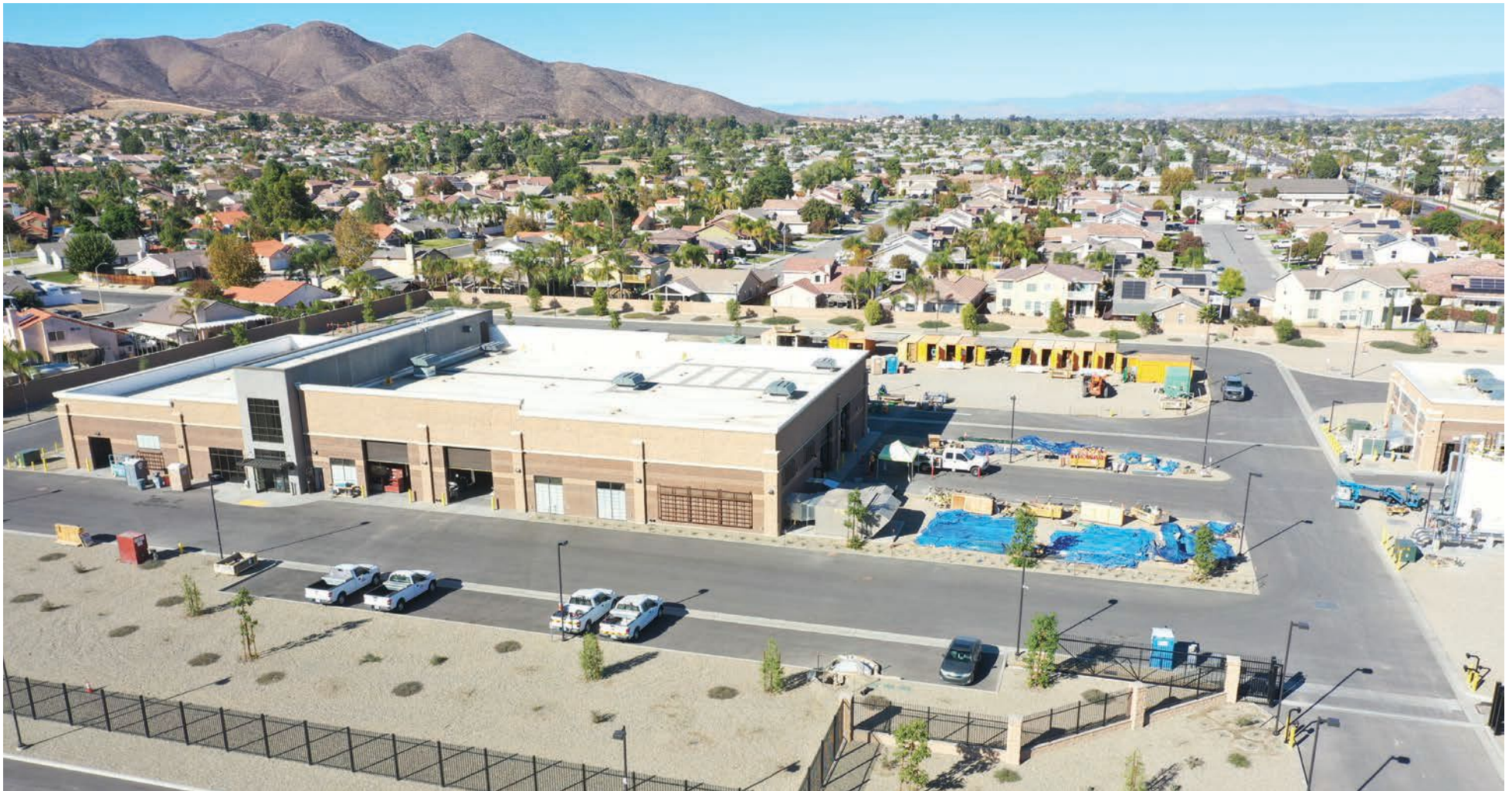
EMWD's Perris II Desalter will be completed in mid-2022, further expanding EMWD's local groundwater desalination efforts as part of a growing portfolio of groundwater projects to enhance local water reliability, improve groundwater quality, and replenish local aquifers.
